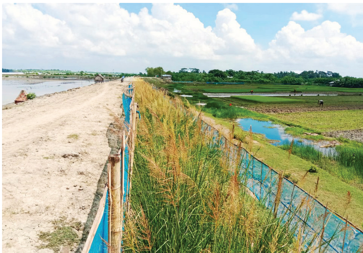
The LoGIC Project promoted the use of vetiver grass as a nature-based solution to reduce soil erosion
