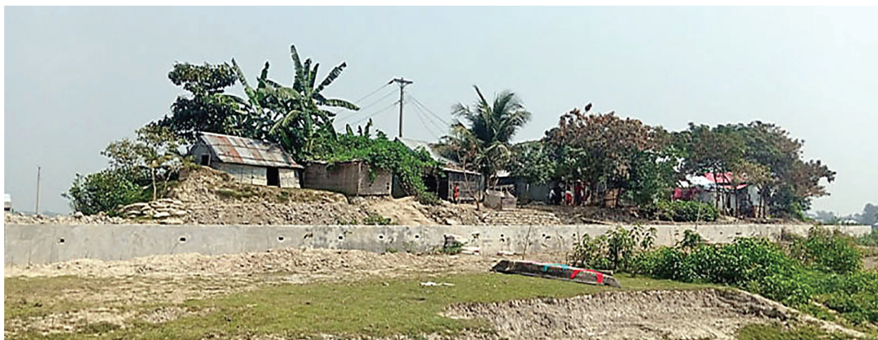
Village protection walls constructed around the base of Hatis in the Hoar areas in Sunamganj reduce soil erosion during flood
