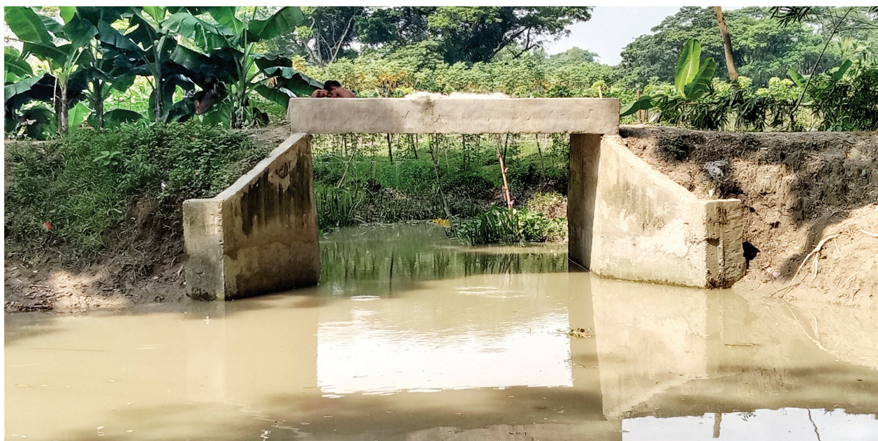
Culvert repaired in Bhola to reduce waterlogging in crop field and human settlement resulting from erratic rainfall
