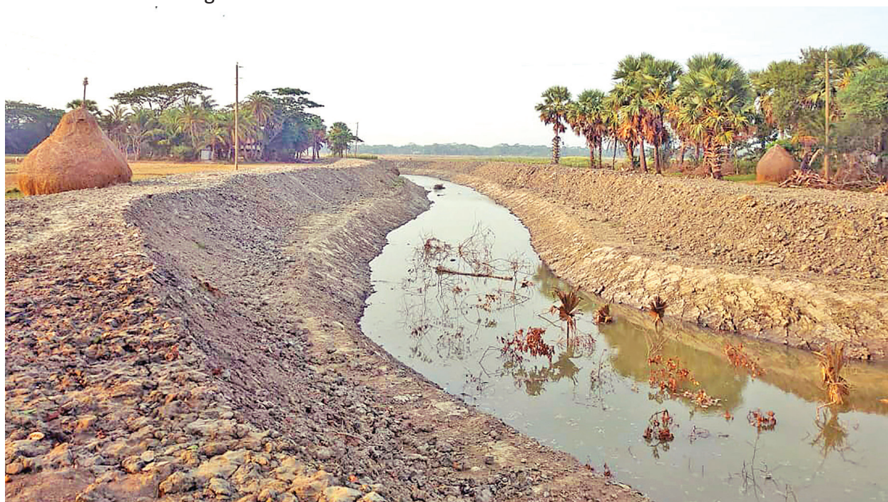
Canal Re-excavated in Barguna with PBCRG to increase supply of surface water for irrigation during the dry season
