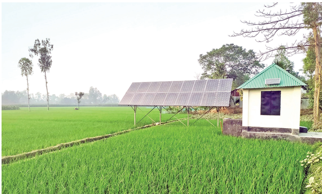
Solar powered plant to irrigate crop field using surface (canal) water in Kurigram
